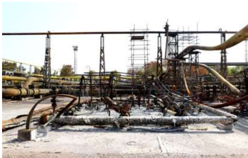
(g). Damaged condensate metering area
