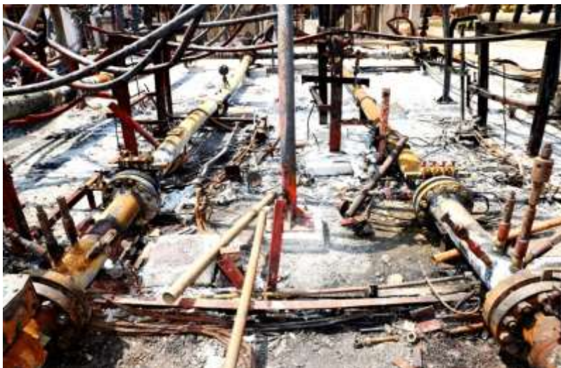
(d). Overview of both meters of condensate pipelines
