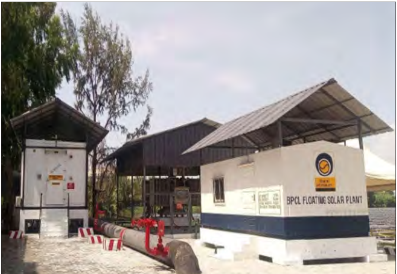
Containerised substation, Transformer and SCADA facility:
